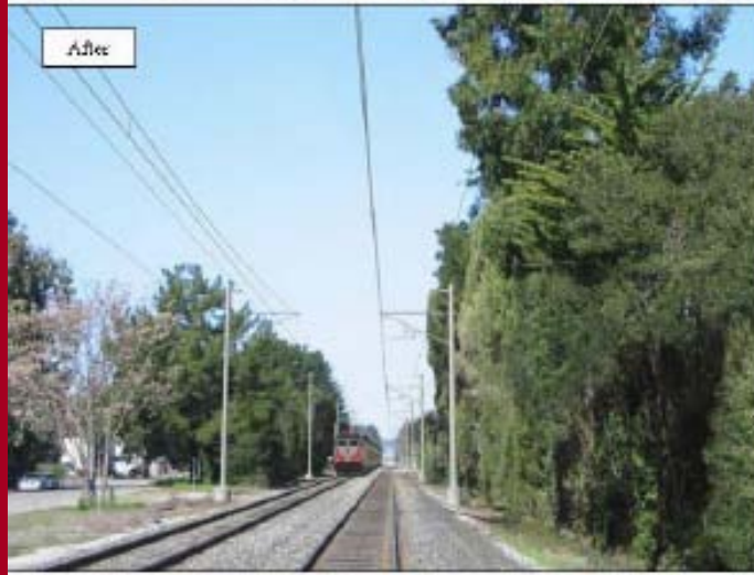
Figure 3.1-1 TREE TRIMMING SIMULATION IN ATHERTON AREA CALTRAIN ELECTRIFICATION PROGRAM
