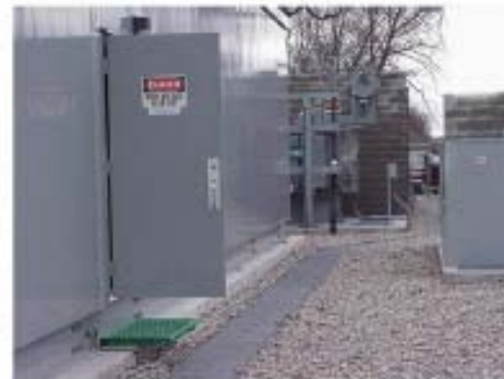
AUTO-TRANSFORMERS WITH FIRE WALLS
