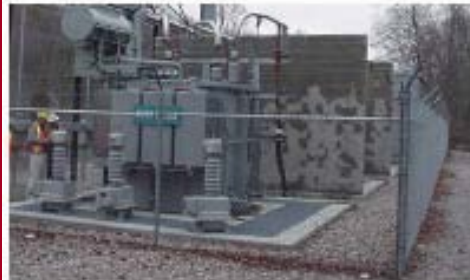
AUTO-TRANSFORMERS WITH FIRE WALLS
